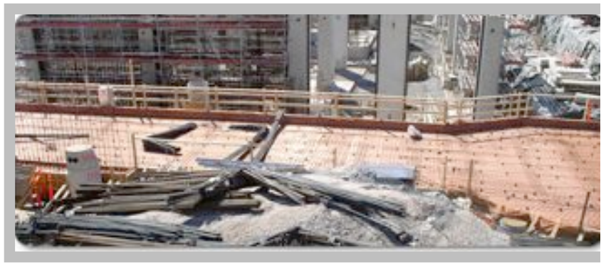
Cuprotect® in foundation, Olkiluoto, Finland/Nuclear plant,
