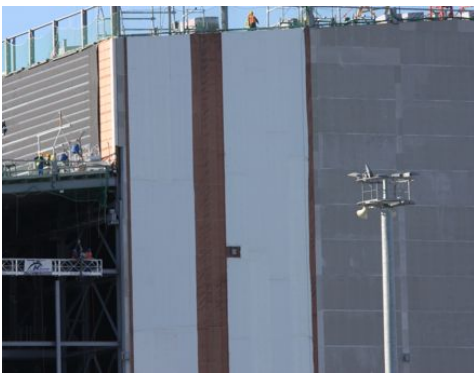
Facade shielding Olkiluoto, Finland/Nuclear plant,
