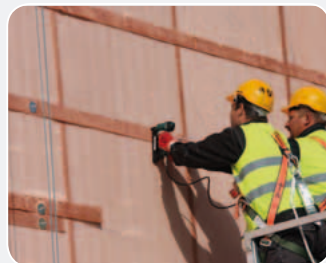
Exterior shielding in a dry construction system
