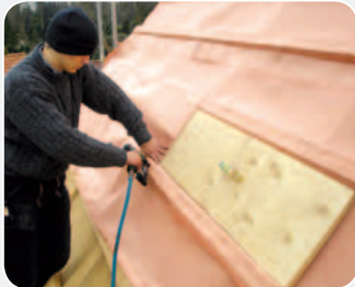
Top roof shielding
