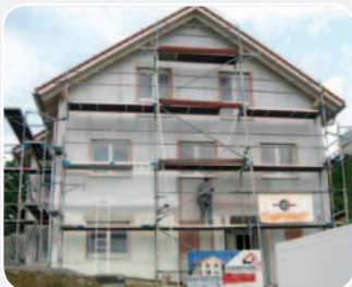
Exterior shielding embedded in ETICS
