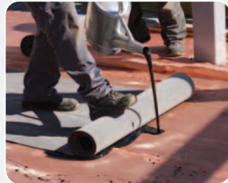
Flat roof shielding with hot bitumen
