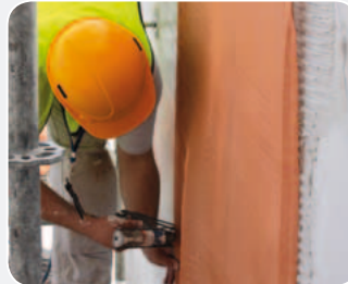
Exterior shielding embedded in plaster
