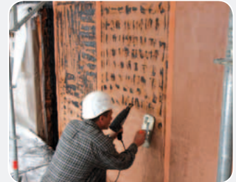
Exterior shielding embedded in hot bitumen
