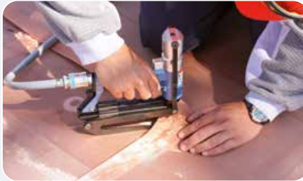
Flat roof shielding
