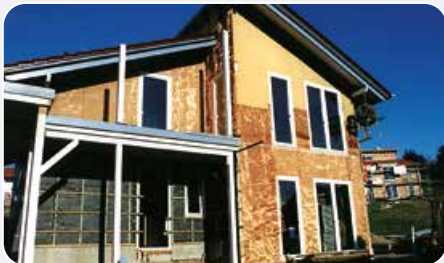
Exterior shielding in a dry construction
