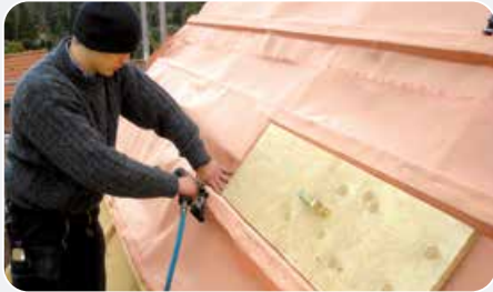
Top roof shielding
